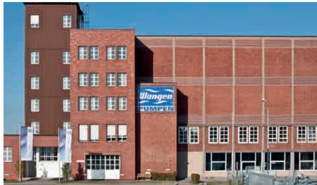
Headquarters building in Wangen, Germany
